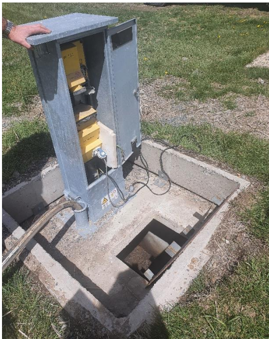
Photo 6 – existing snowmaking pit requiring drainage
